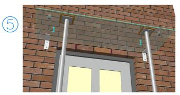
Remove pre-assembled fixings from the brackets. Sit glass onto the brackets and re-assemble the fixings through glass and both brackets.
